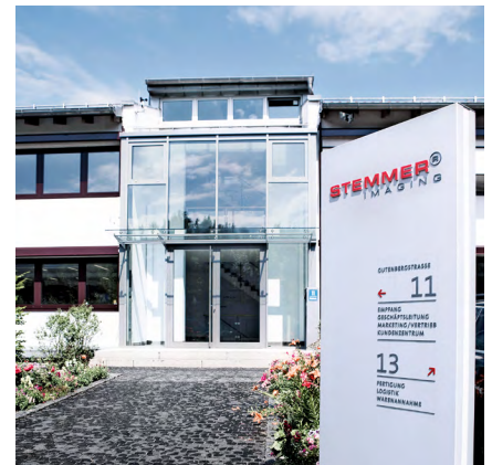
Headquarters in Puchheim
